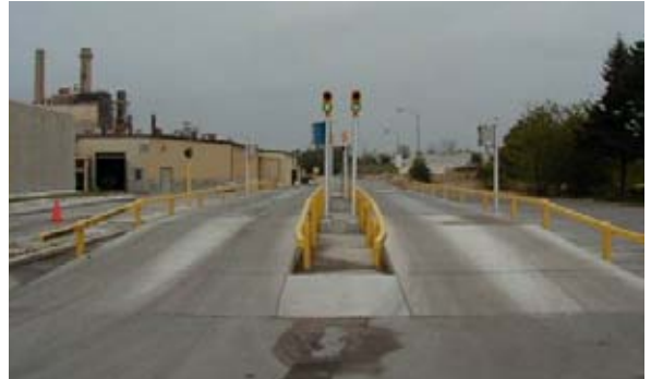
Scale-mounted guiderails are attached to the side of the weighbridge modules with bolts or welded brackets
