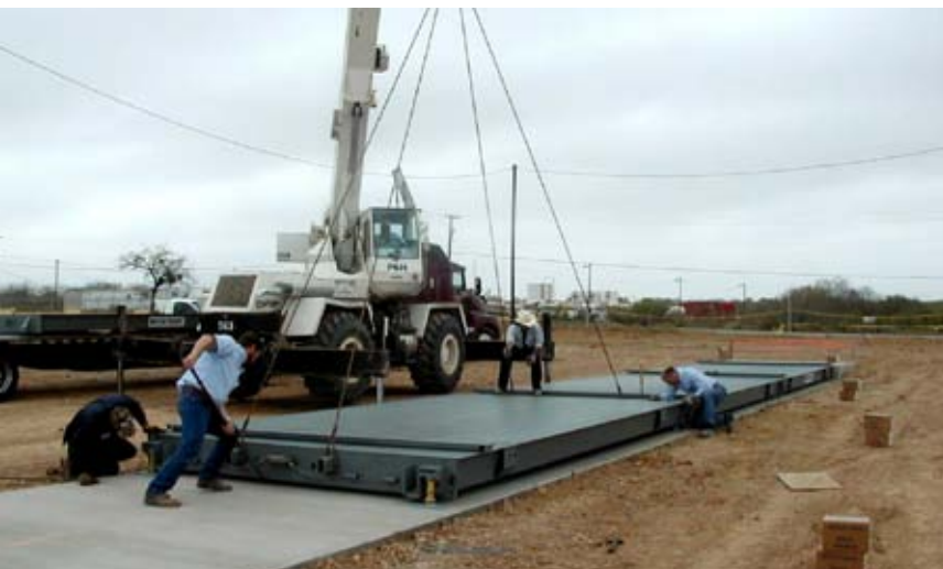
A steel deck weighbridge is installed
